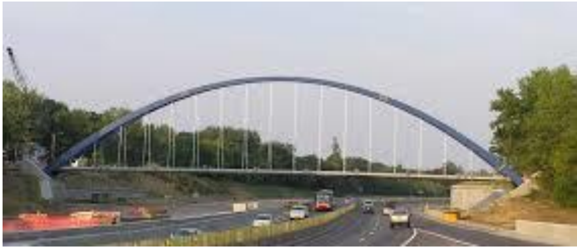
Figura 19 Griffin Memorial Bridge
