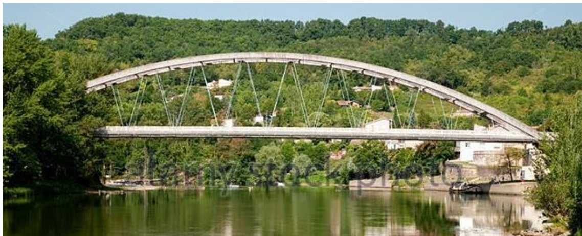
Figura 20 Castelmoron Bridge Francia 1933
